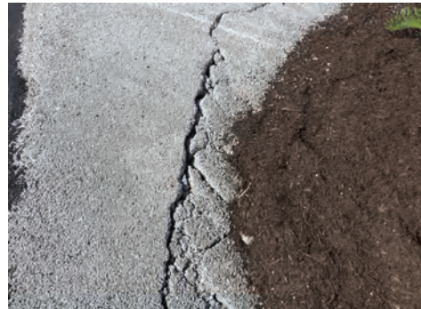
7 CRACKING-STRUCTURAL
