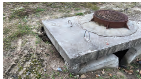
19 OUTLET STRUCTURE EROSION
