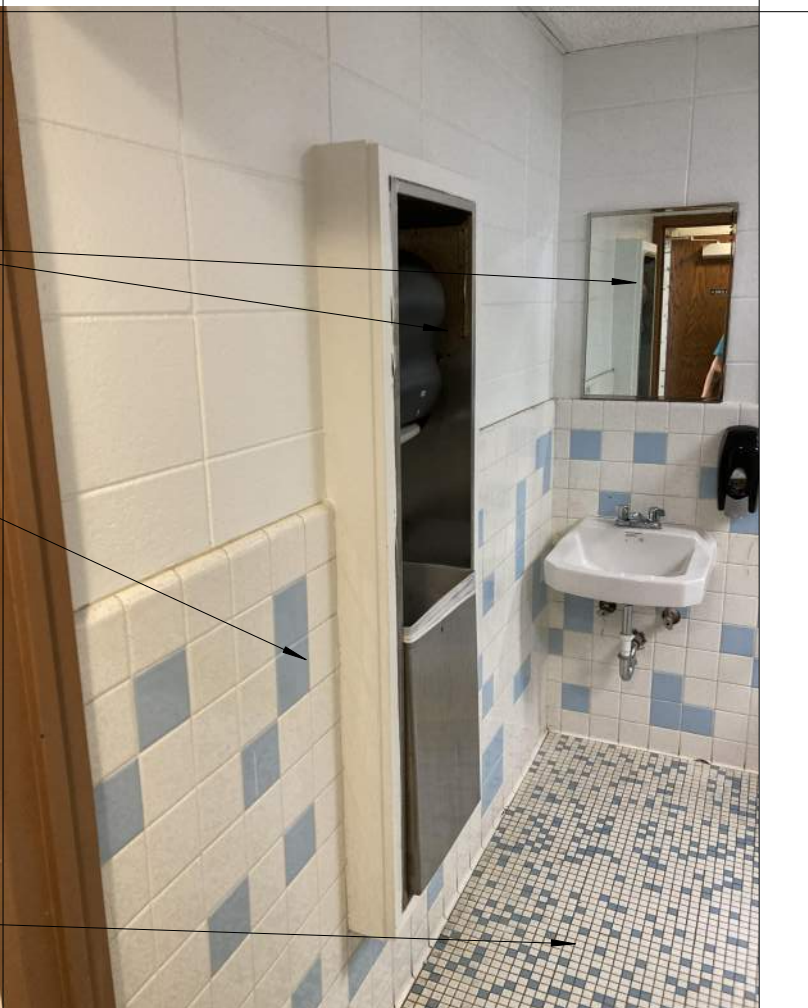
2.6 EXISTING BATHROOM ACCESSORIES
