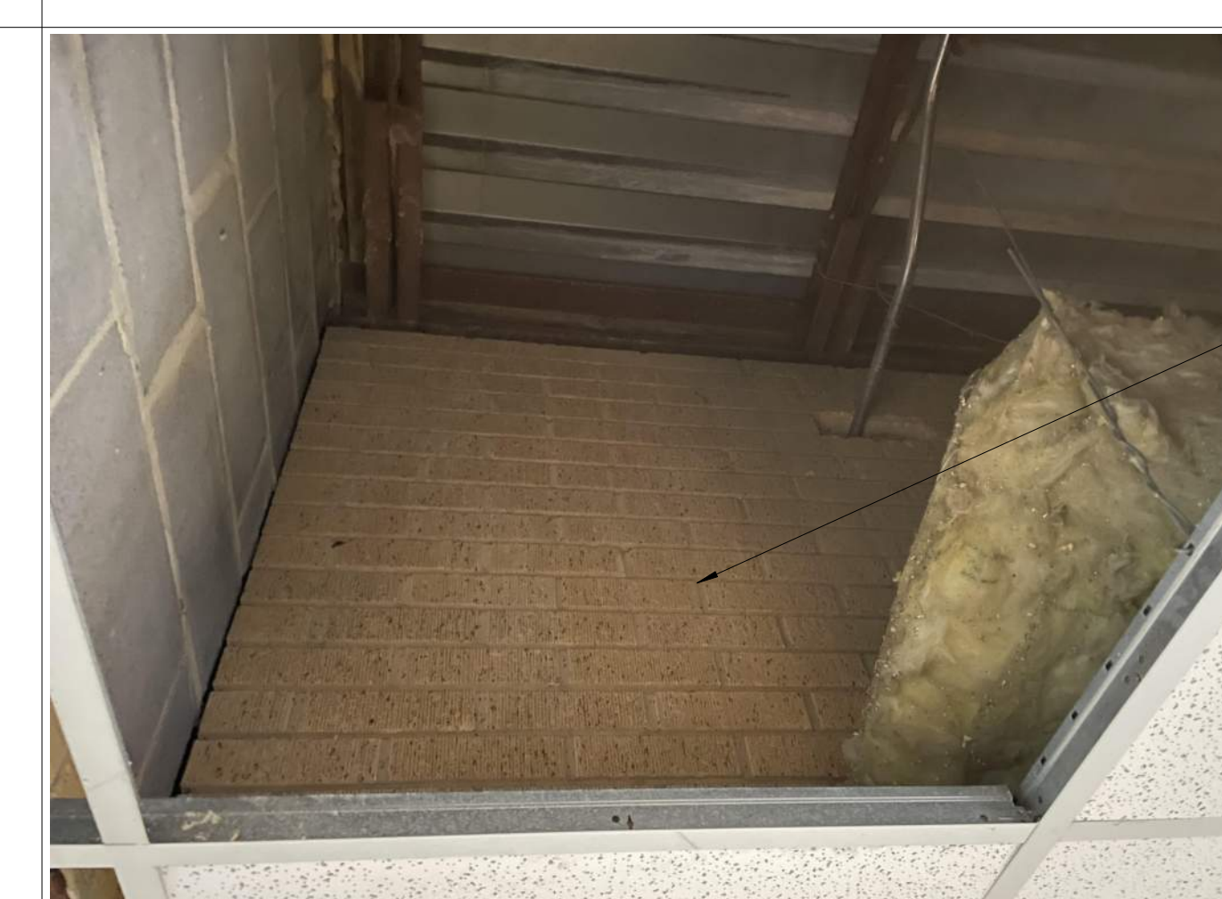
2.16 EXISTING LOAD BEARING WALL ABOVE CEILING
