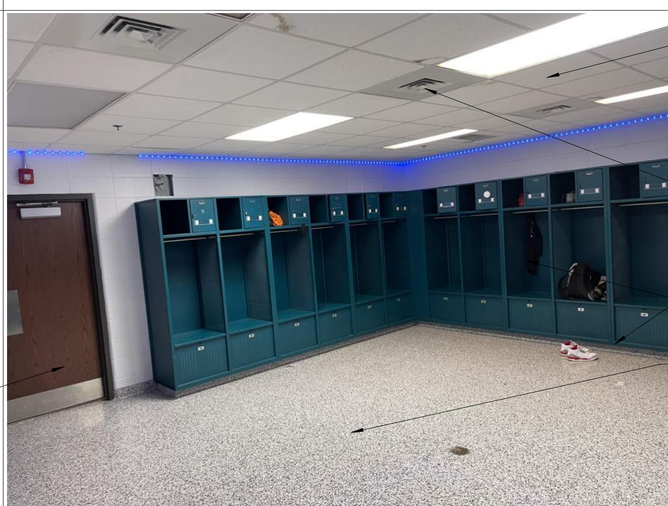
2.11 EXISTING LOCKER ROOM
